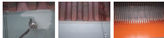
During NEOGUARD TOUGHNESS GRAY application After NEOGUARD TOUGHNESS GRAY application After NEOGUARD TOUGHNESS RED OXIDE application
