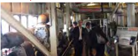
In the engine room, steam pistons are on the left, while on the right are steam condensers.
